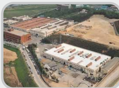
• Hwaseong 1 st Plant
