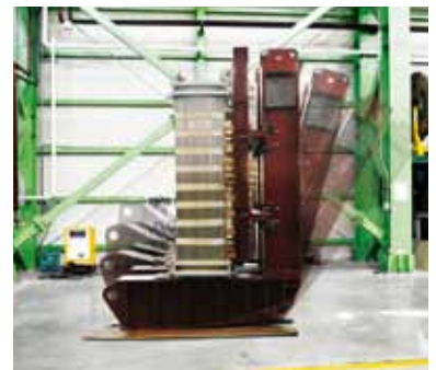
· ERECTION OF CORE ASSEMBLY
