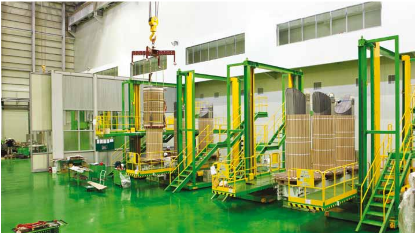
· CORE AND COIL ASSEMBLY SHOP
